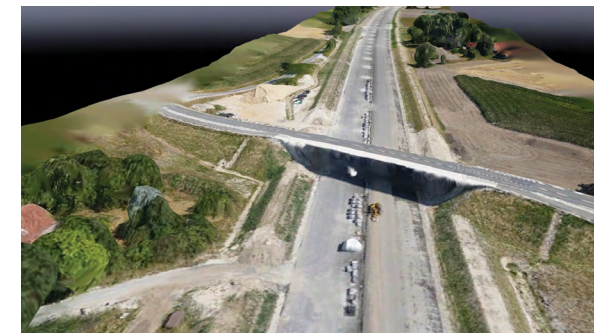
Above: From the Real World to a 3D Pointcloud: Easy workflow thanks to direct georeferencing helped the team rapidly collect data to generate a 3D pointcloud of the 12km stretch of Autobahn.
